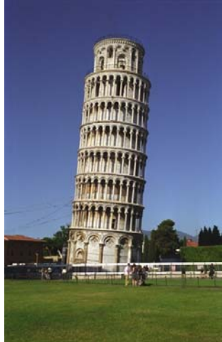
Leaning tower of Pisa
