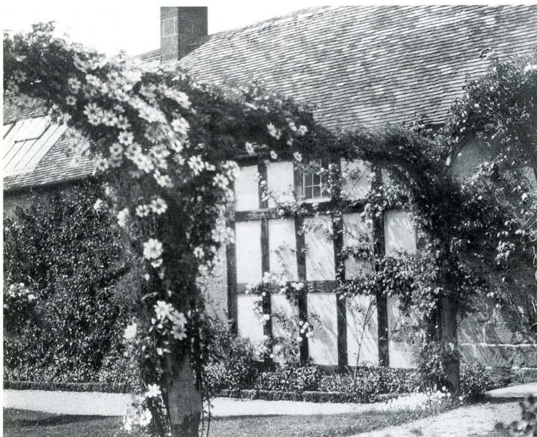
Cottage with roses: its character is given by its dominant centers, the roses, the arch of roses, the timber frame, the plaster squares.
