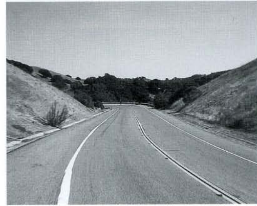
Road cut through the hills
