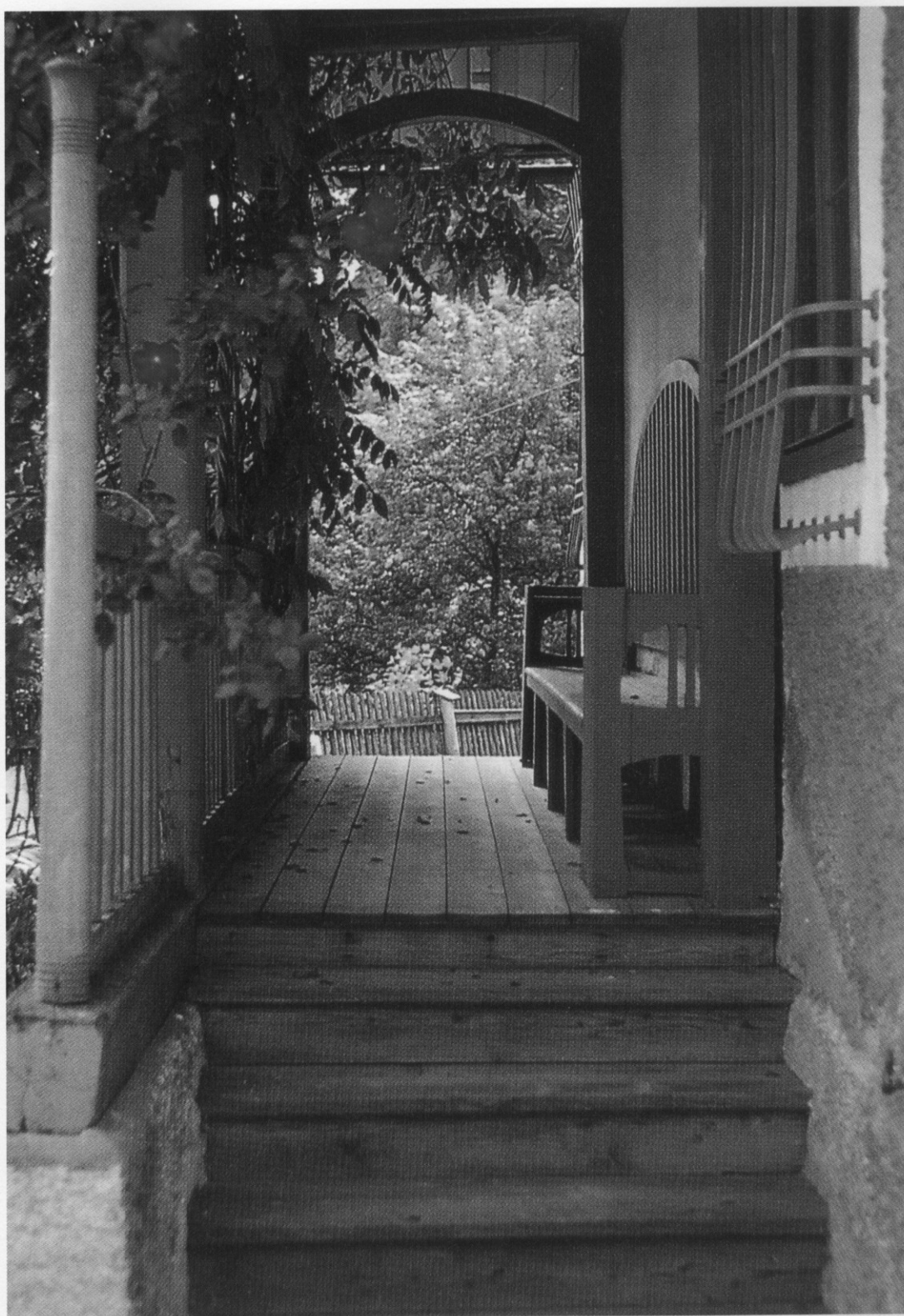
Recursive character of living structure, visible in a front door stoop
