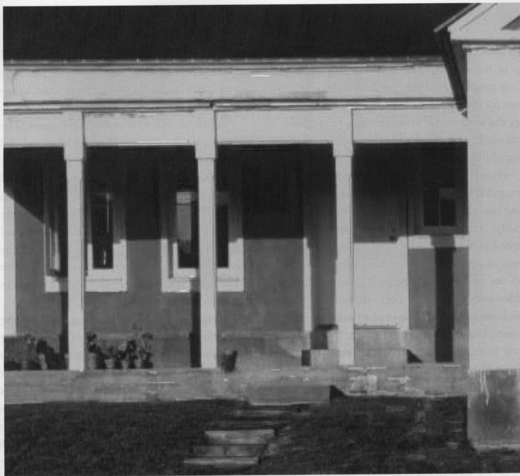
An example of a highly modern cast concrete construction, in which the columns, and the column-bases, are brought to life. The Martinez house, California, by Christopher Alexander, 1984.
