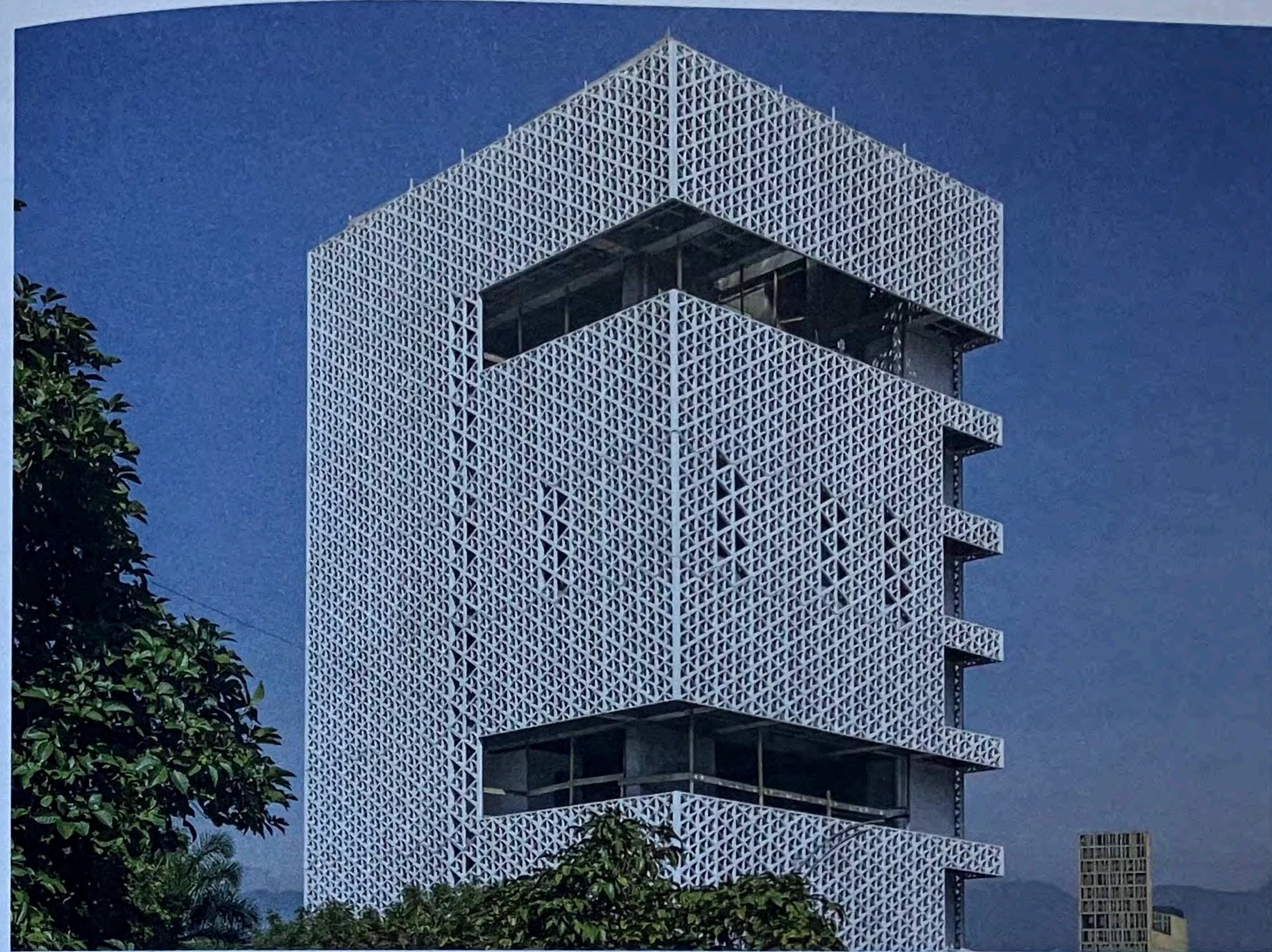
Fig. 2: The exterior shading screen is made from prefabricated Glass-fibre Reinforced Concrete (GRC). A single-glazed facade will be fitted behind the screen, on the interior side. The lack of HVAC infrastructure means double or triple glazing is unnecessary.
